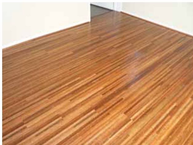
An engineered cocowood floor in service.
