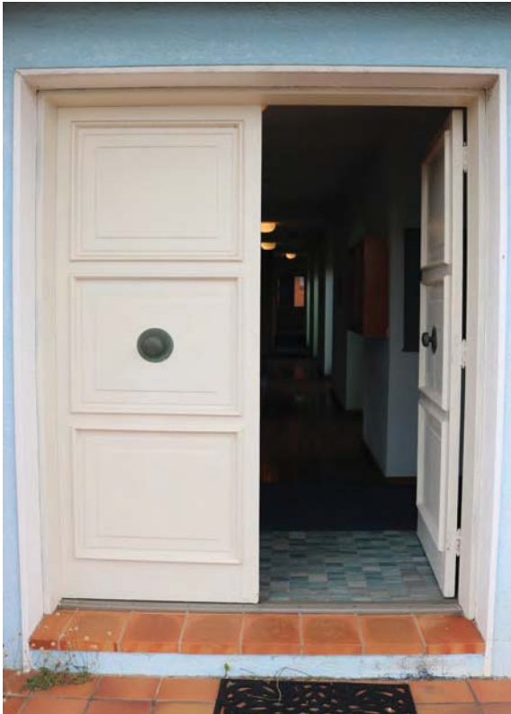
Figure 5: Front doors (Queensland Government, 2021.)
