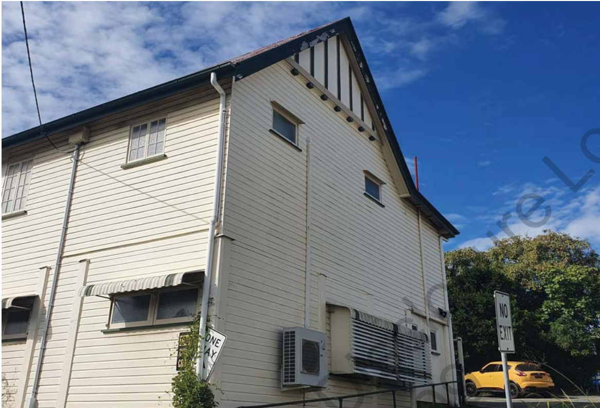
Figure 11: Southwest end of Hall (Queensland Government, 2021.)
