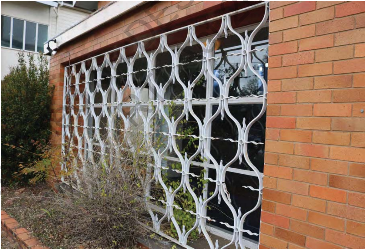
Figure 7: Metal screen to lobby window (Queensland Government, 2021.)
