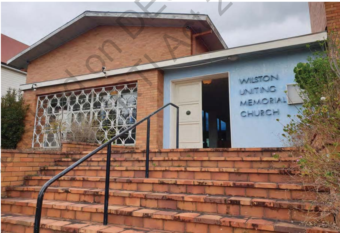
Figure 4: Entrance from Hawdon Street (Queensland Government, 2021.)
