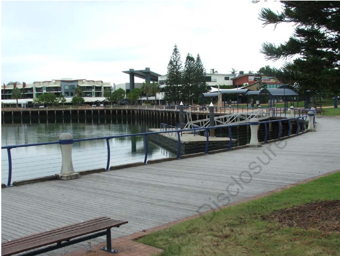
Photo 3 – Taken from park looking towards boardwalk (foreground) council owned temporary mooring facilities (midground) and site of proposed lease (water in background)
