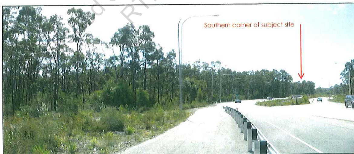
Figure 13– View towards the site from the northern side of Eenie Creek Bridge.
