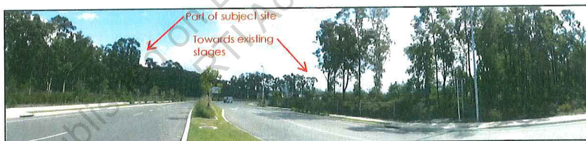
Figure 4 - View into Shire Business Centre from roundabout to north-east of the site.
