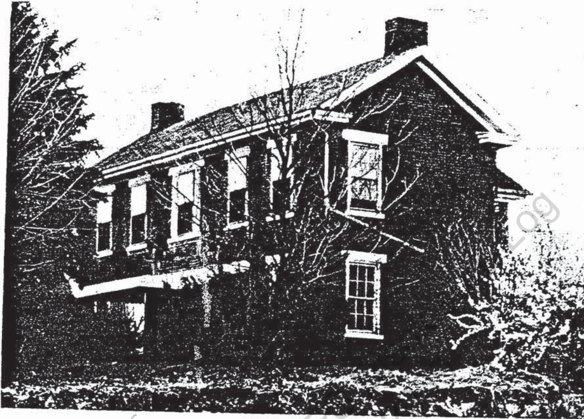
Figure 27.—Test structure 51, near a coal mine.
