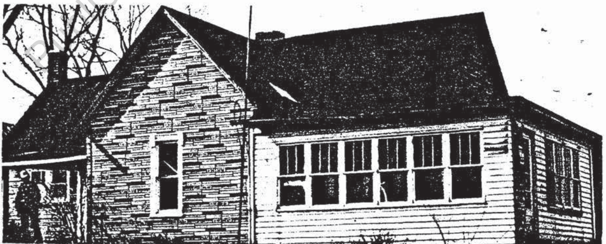
Figure 21.—Test structure 27, near a coal mine.
