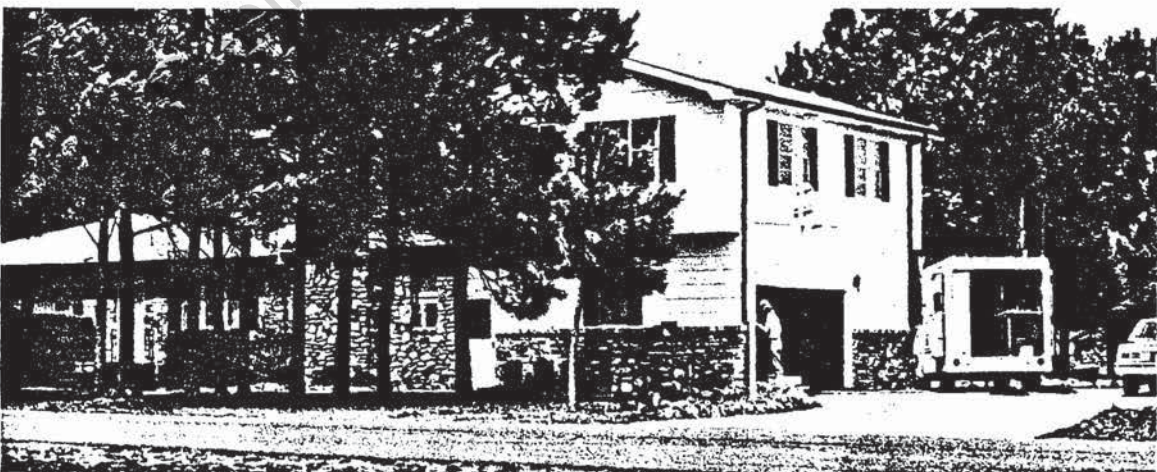
Figure 18.—Test structure 22, near a quarry.
