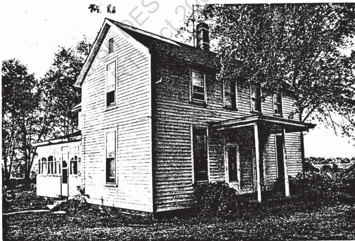
Figure 15.—Test structure 19, near a coal mine.
