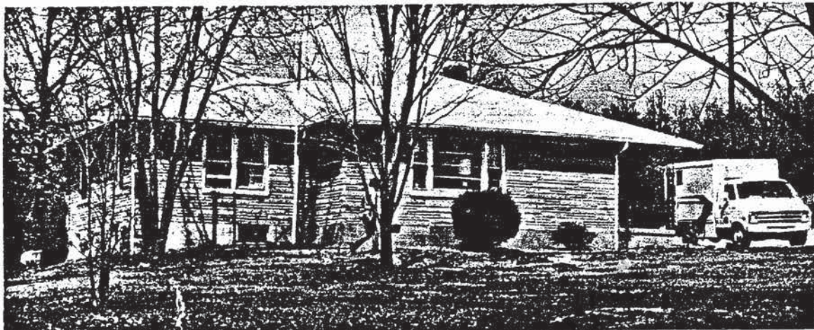
Figure 24.—Test structure 30, near a coal mine.
