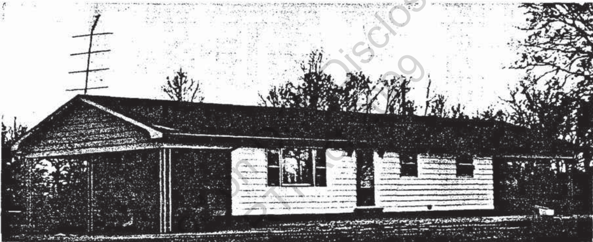
Figure 17.—Test structure 21, near a coal mine.
