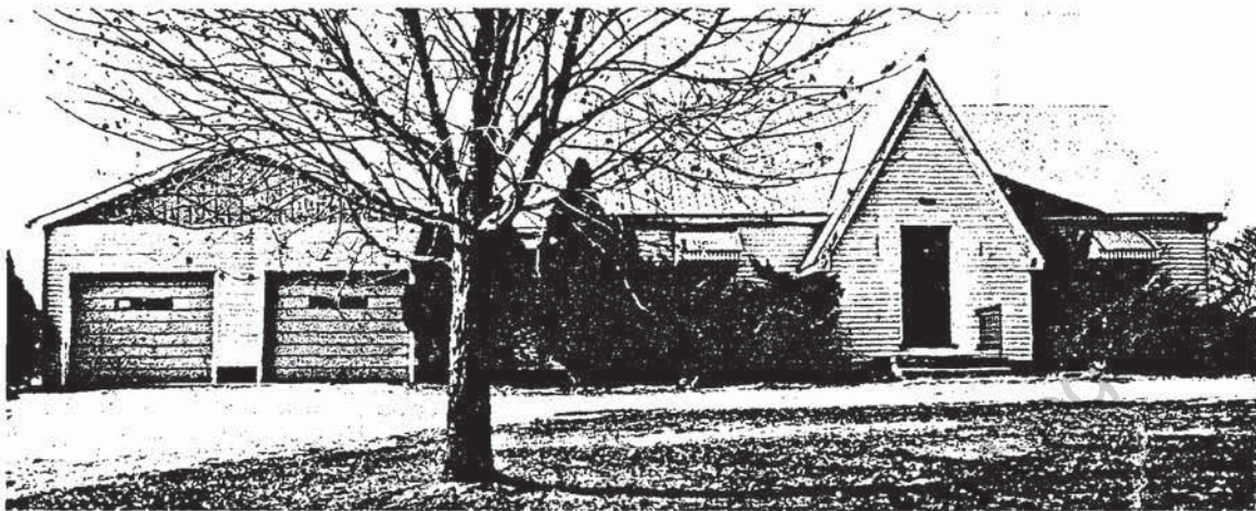
Figure 16.—Test structure 20, near a coal mine.
