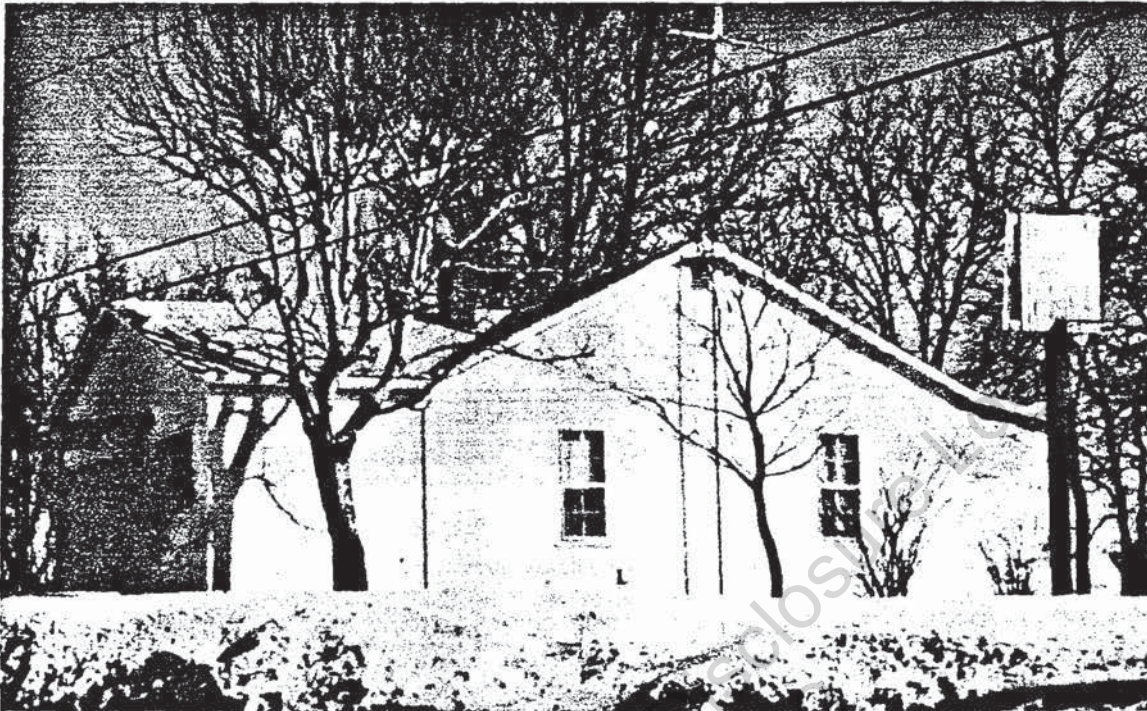
Figure 22.—Test structure 28, near a coal mine.
