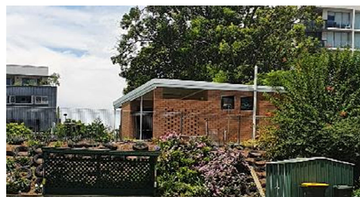
Figure 14. Northern side of larger associated outbuilding.
