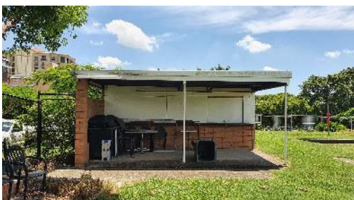
Figure 13. Southern side of larger associated outbuilding.
