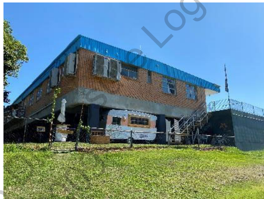
Figure 6. Northern side of building.
