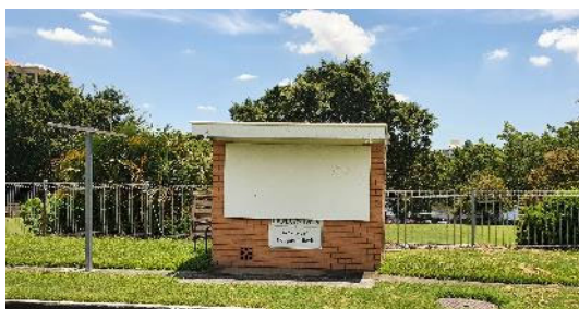
Figure 9. Southern side of smaller associated outbuilding.
