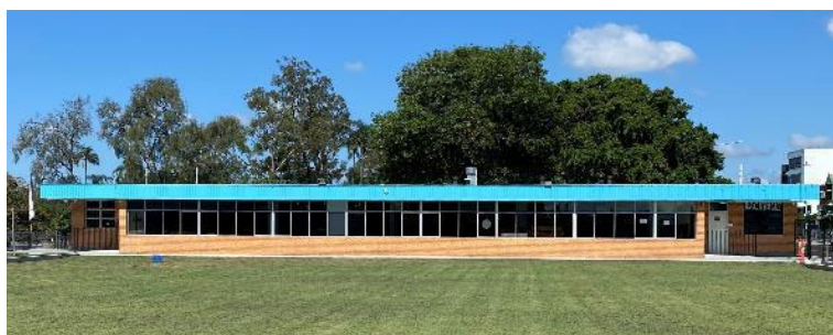
Figure 2. Western elevation of former East Brisbane Bowling Club building fronting the bowling green – the front of the building.
