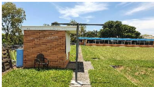
Figure 11. Western side of smaller associated outbuilding.
