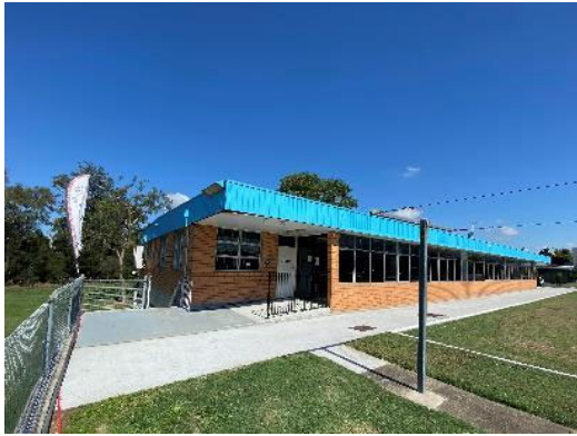
Figure 3. North Western corner.
