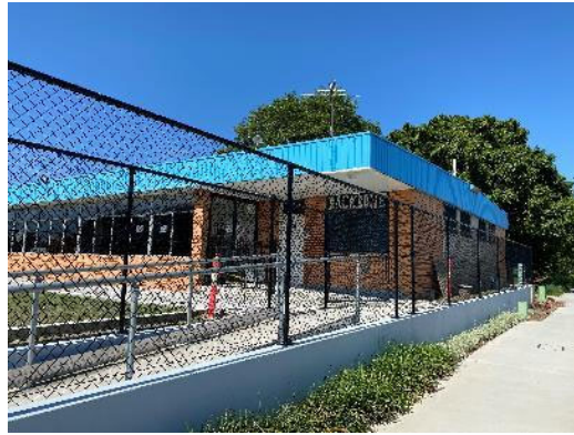
Figure 4. South Western corner near Lytton Road.
