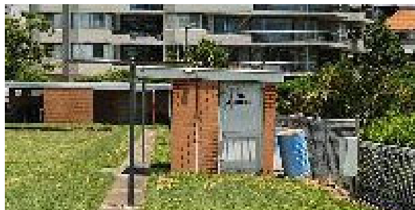
Figure 10. Eastern side of smaller associated outbuilding.
