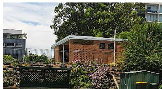
Figure 14. Northern side of larger associated outbuilding.
