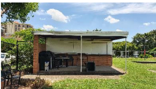
Figure 13. Southern side of larger associated outbuilding.
