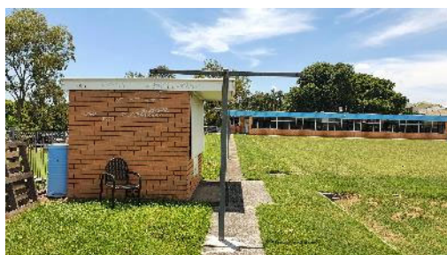
Figure 11. Western side of smaller associated outbuilding.
