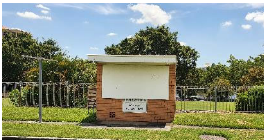
Figure 9. Southern side of smaller associated outbuilding.
