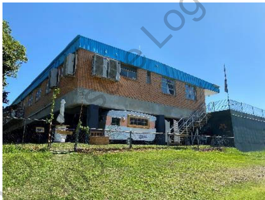
Figure 6. Northern side of building.
