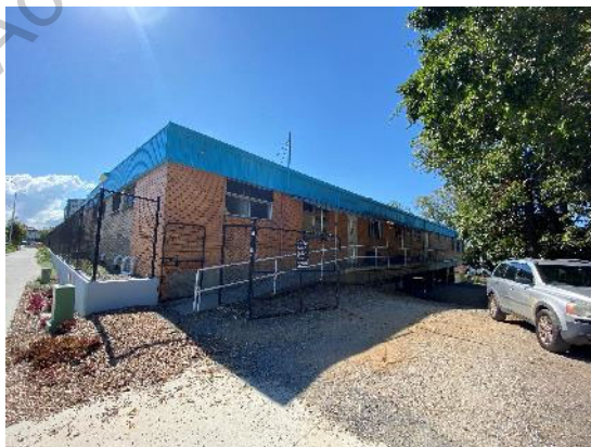
Figure 8. South Eastern corner of building showing ramp access to rear of building.
