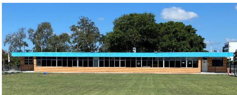
Figure 2. Western elevation of former East Brisbane Bowling Club building fronting the bowling green – the front of the building.
