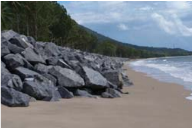
Plate 3. Hard structures, such as this rock wall at Clifton Beach near Cairns, have been commonly used to control shoreline erosion.
