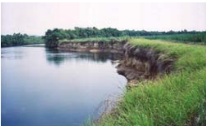
Before erosion control works
