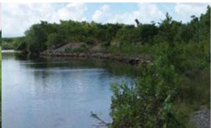
After erosion control works
