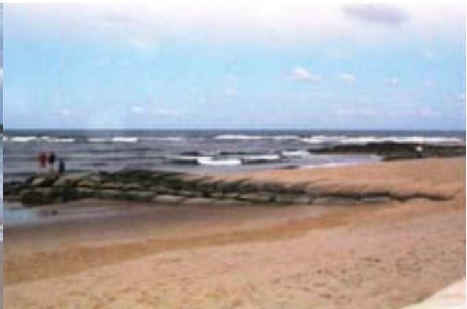
Plate 4. A groyne made of geotextile bags, Cottontree Beach, Maroochydore.
