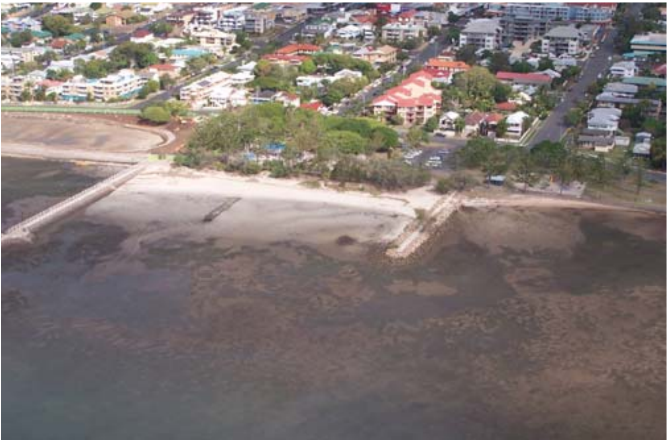
Plate 1. Placement of sand on the soft-sediment foreshore of Pandanus Beach, Wynnum, Moreton Bay, commenced in the late 1980s. (Note: Placement of sand at this site is consistent with the policy due to historic disturbance through sand placement.)
