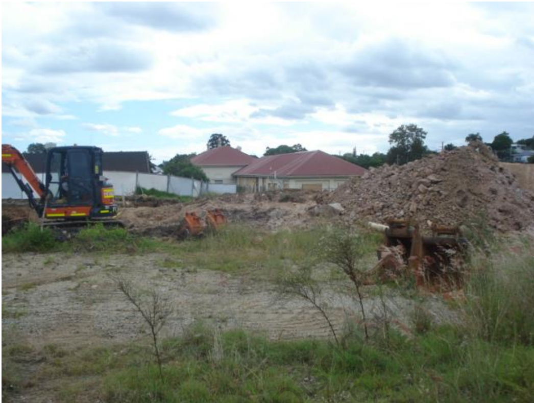
Plate 3 – Overview portion of the Site (facing west).
